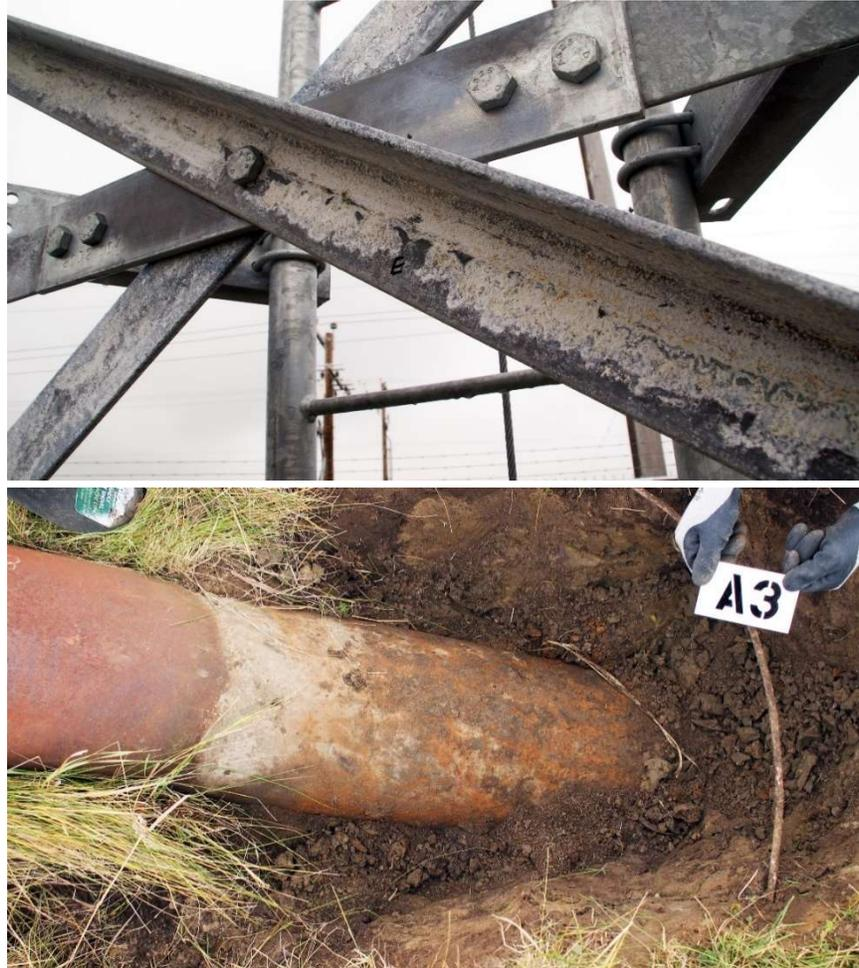
**Figure 1: Sample photos of above-grade and below-grade corrosion at telecom towers**
