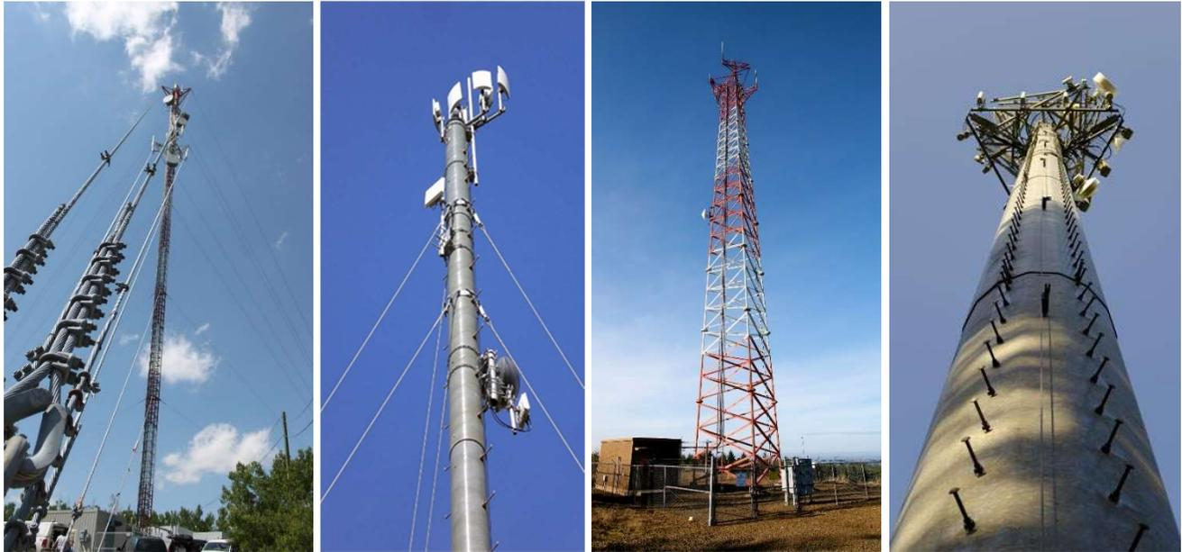
**Figure 2: Different types of communication towers**
