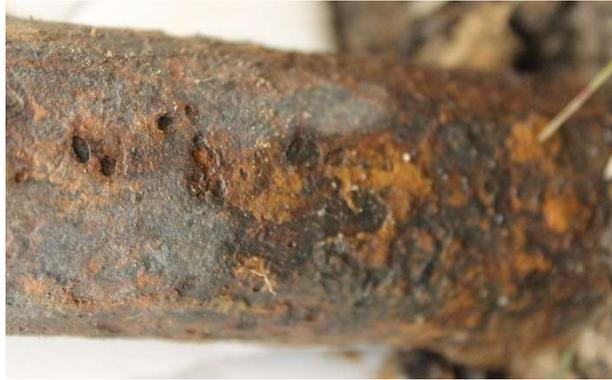
**Figure 7: Sample photo of MIC at anchor shafts of a telecom tower**
