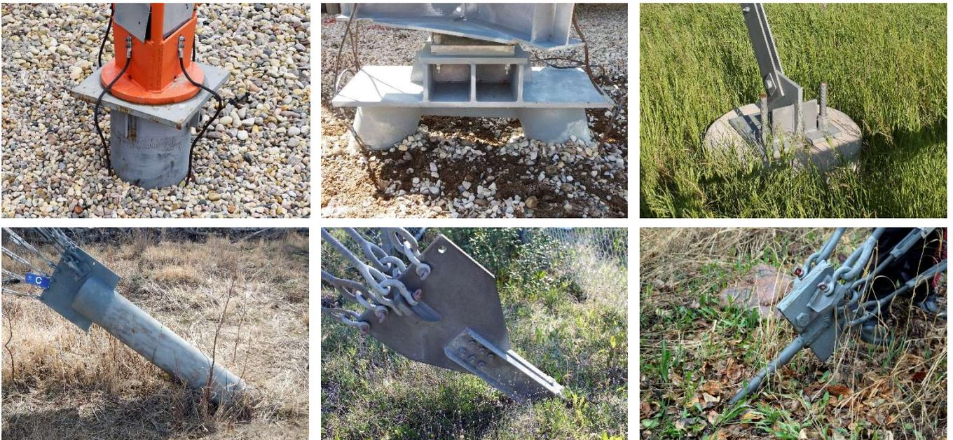
**Figure 3: Sample photos of foundation designs at base and anchor footings**
