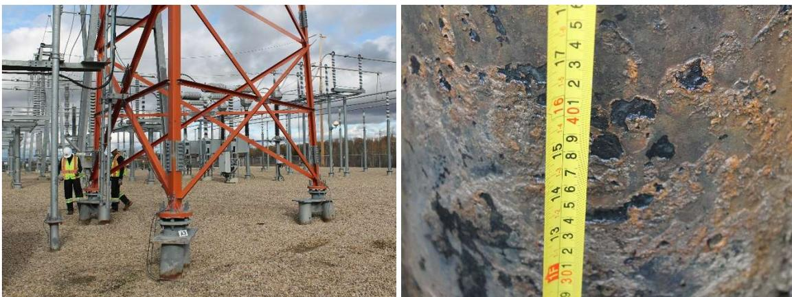
**Figure 8: Galvanic corrosion at screw-pile foundations of a telecom tower located inside a substation**
